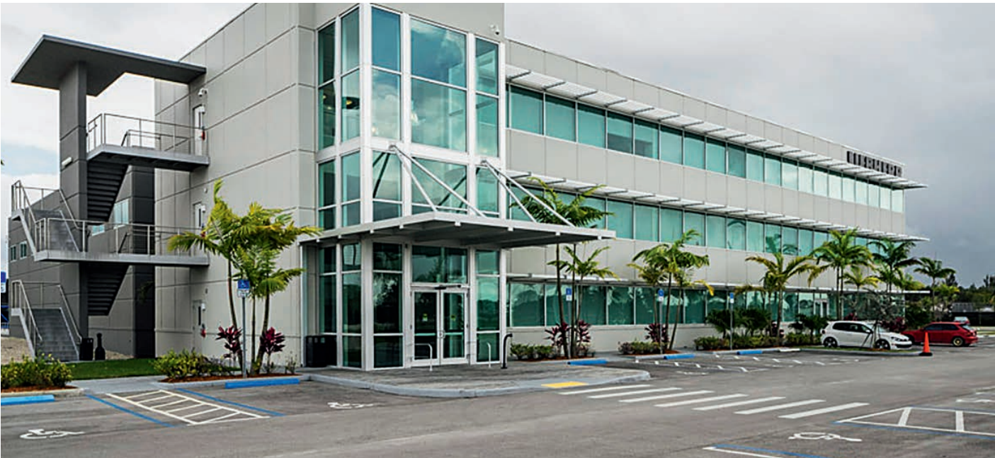
Liebherr offices in Miami, Florida, USA
